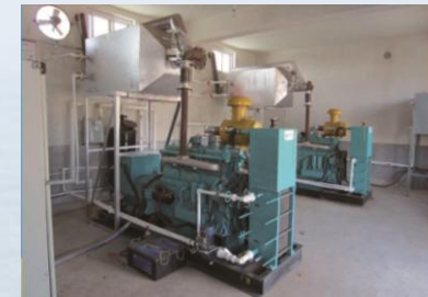
20kW, Two Biogas generator sets with CHP, Henan China
