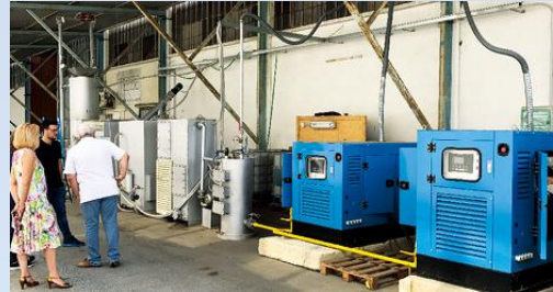
50kW, Gasification system, MARCON Italy
